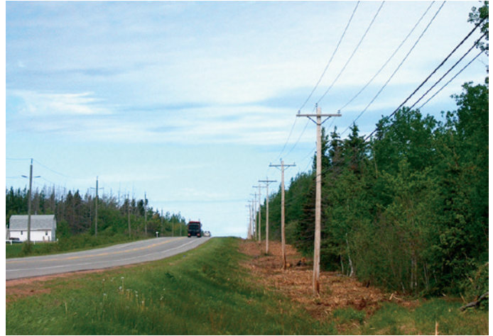
Vegetation and trees have been cleared from power lines to ensure correct distance and safety requirements are in place.
