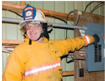
Miles Boulter, Chief Training Instructor for the P.E.I. Firefighters Association Fire Training Centre, demonstrating how to open main switches in buildings.
