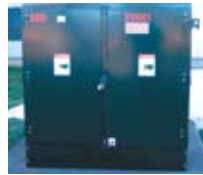
Padmounted Transformer
