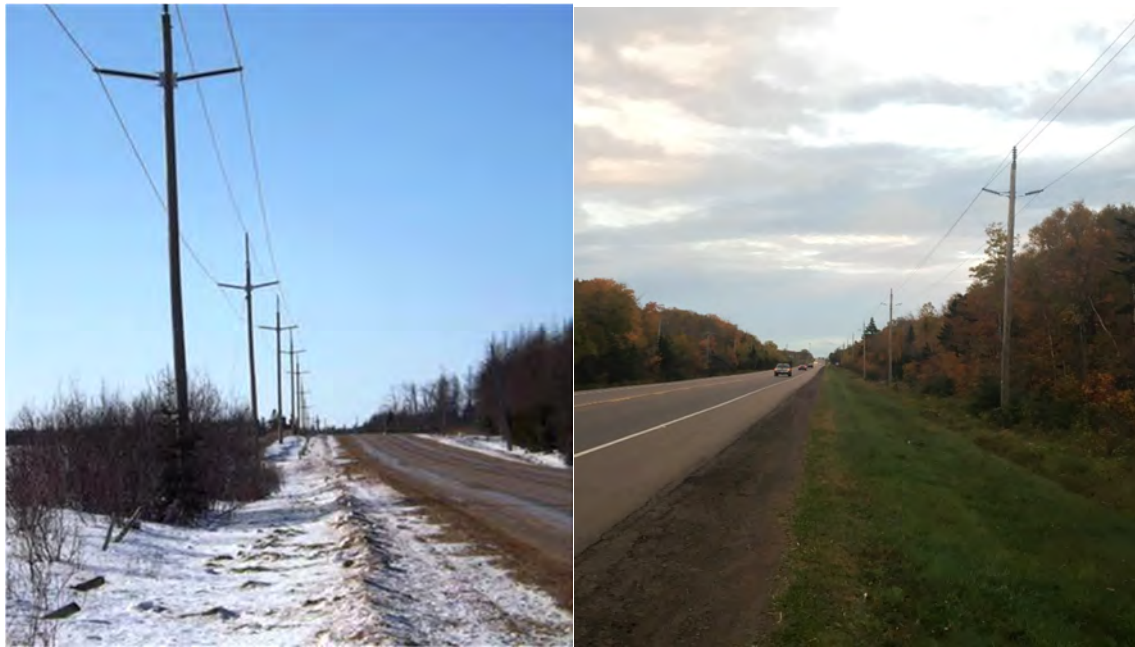
Photo 1 Typical 138-kV transmission line construction along a public road in PEI (left) and T-3 69-kV transmission line construction along the Trans-Canada Highway (right) (photos courtesy of Maritime Electric)
